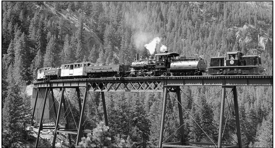
Crossing the Devil's Gate bridge over Clear Creek. – Photo © 2005 Bruce Nall.
